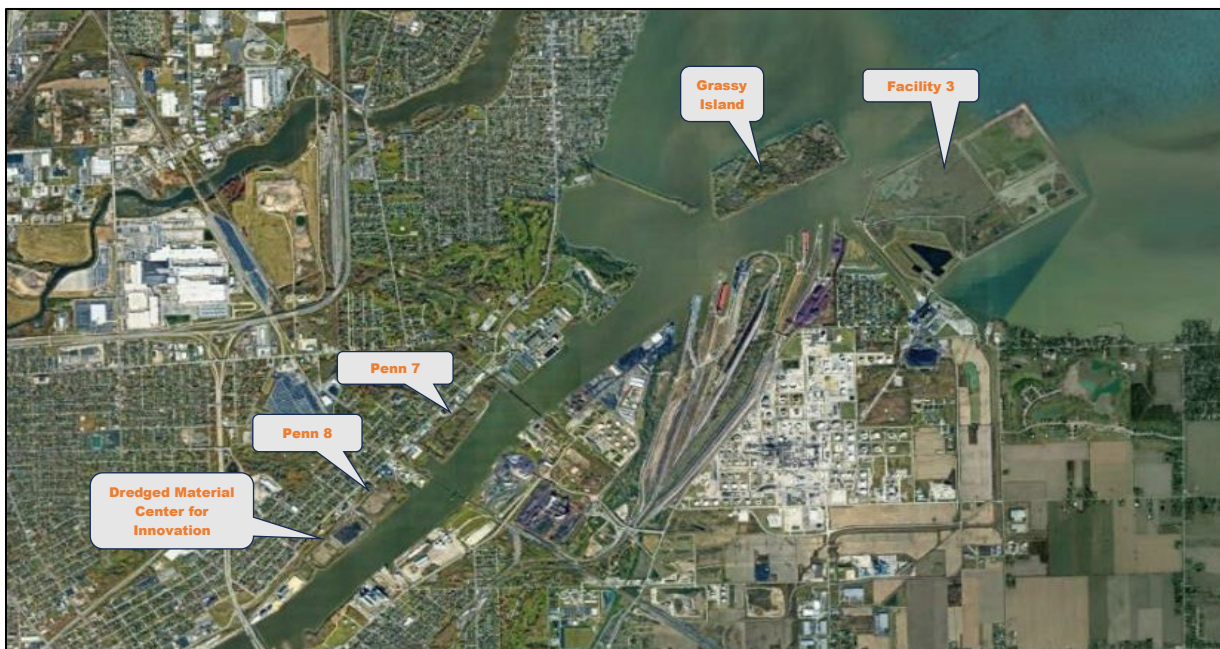
Figure 17. Overview of the confluence of the Maumee River with Maumee Bay showing the Port of Toledo docks and several of the former and current CDFs. Base image courtesy of Google maps-2024.
