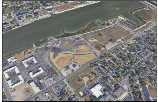
Figure 15. Glass City Metropark. Phase 1 was completed in 2019. This image shows Phase 2 under construction in 2021.
