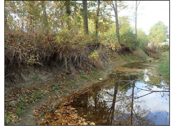
Undercut bank at the upstream end of the site
