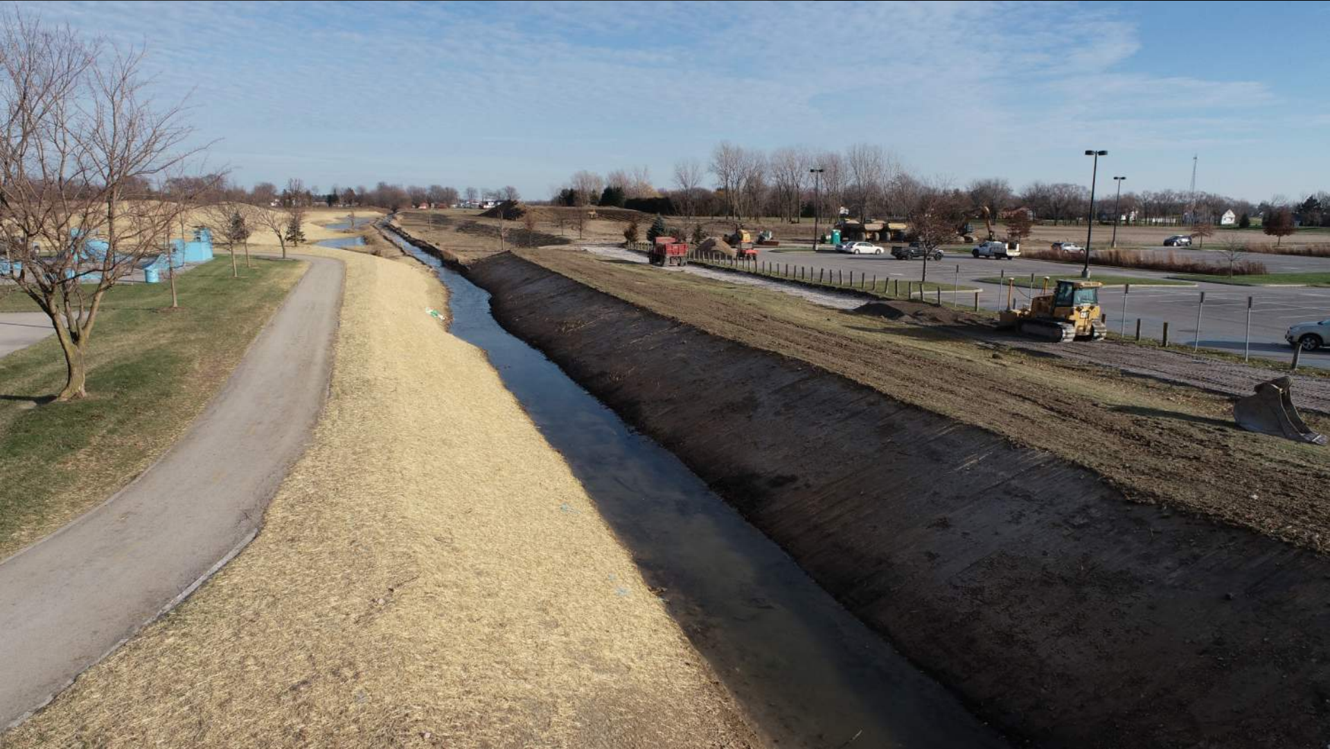
Streambank Regrading and Stabilization, Wolf Creek Stream and Floodplain Restoration Project, December 2023
