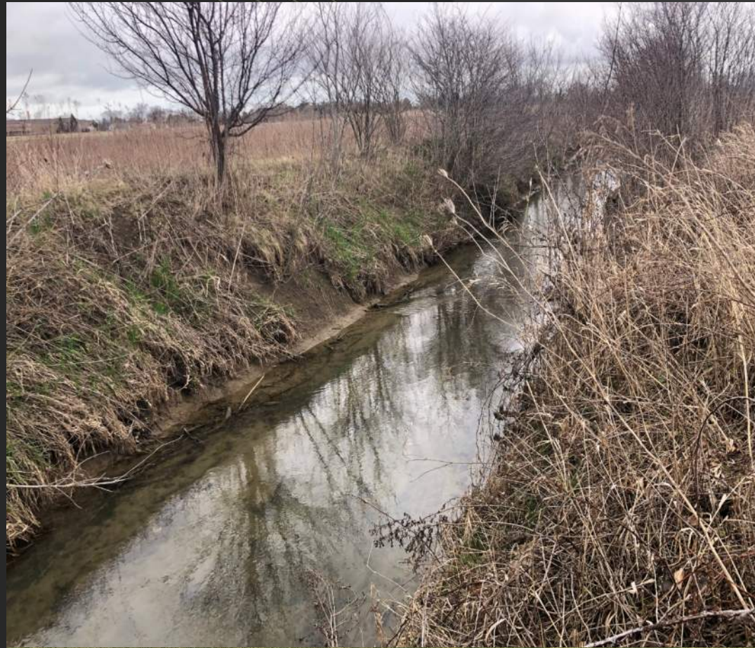
Channelized and steep banks, Wolf Creek flows through the City of Oregon's Recreation Complex, located off of Starr Avenue Extension
